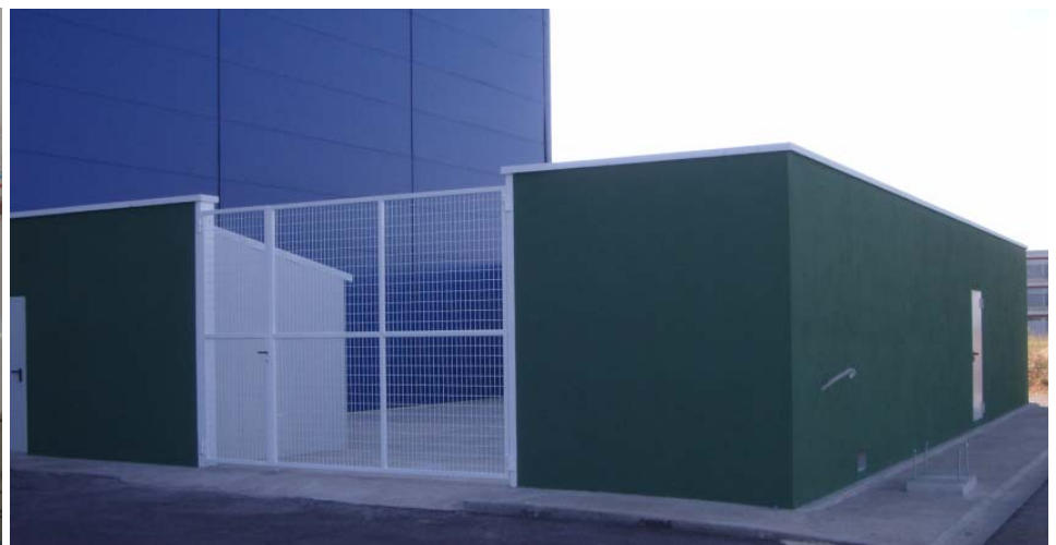
Illustration 10 – Hydrogen refuelling station area
