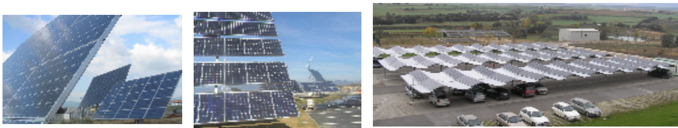
Picture 1 – Photovoltaic grid Installation.
