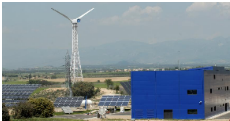
Picture 6 – Aragon Hydrogen Foundation Research Center
